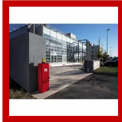
Electromechanical Boom Barrier
